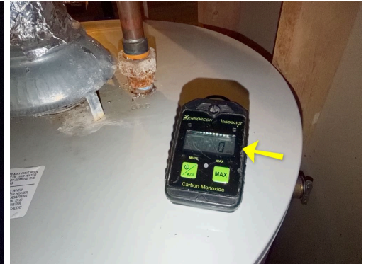
No elevated carbon monoxide readings during inspection near water heater
