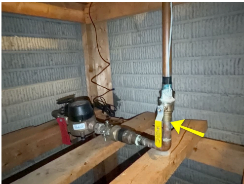
Front wall of utility room
