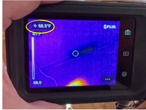
Return air temperature
