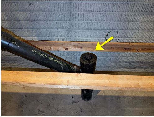
Front wall of utility room
