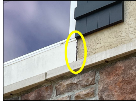
Pain maintenance needs to wood frame windows
