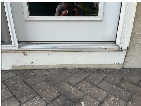
Rear patio door kickplate needs repainted
