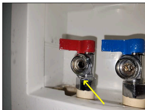
Supply valve leaks
