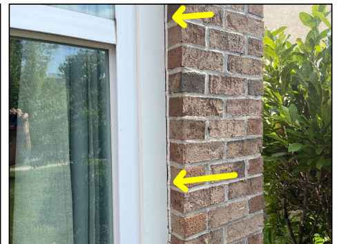
Caulking needed to front windows
