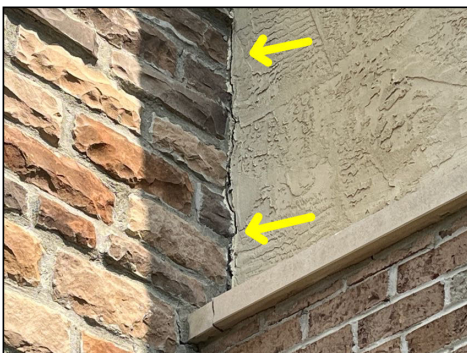
The siding is lacking proper sealant joints at intersections (Brick meets stucco)
