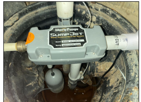
Waterpowered back up system
