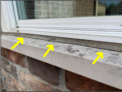
The front dining room window sill mortar, shows evidence of cracking.
