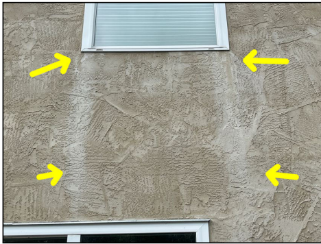
Minor cracking and staining of the stucco exterior walls at (rear below windows).
