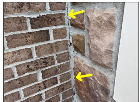
Cracked brick mortar requires repair
