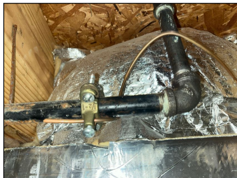
The CSST gas piping appears to be bonded as recommended.
