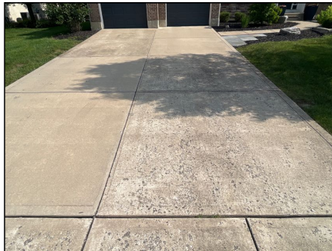
Driveway surface deterioration observed
