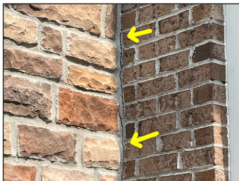
Cracked brick mortar requires repair
