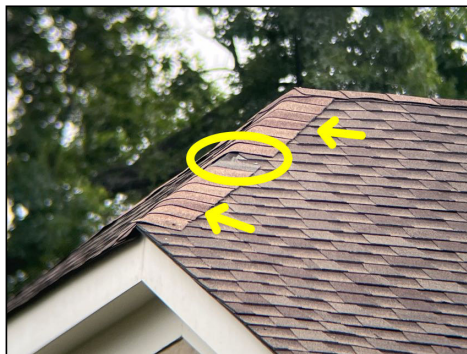
Wind damaged and missing shingle observed at (front Southwest corner)
