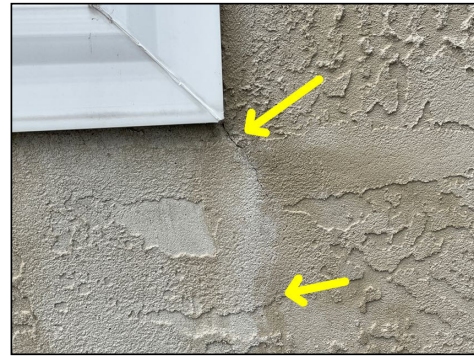
Cracking and water stains of rear stucco wall below windows
