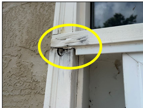
Exterior door frame at top left corner shows signs of wood rot (Rear patio door)
