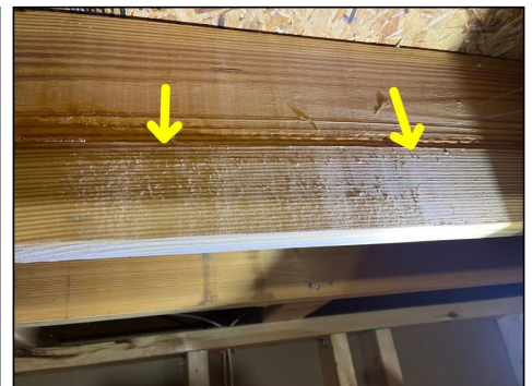
What appears to be possible mold growth (front basement unfinished storage room)
