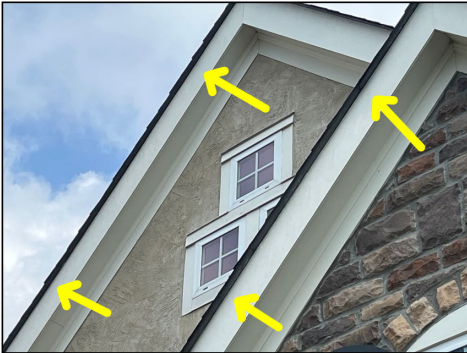
Missing drip edge flashing is not required but is recommended.
