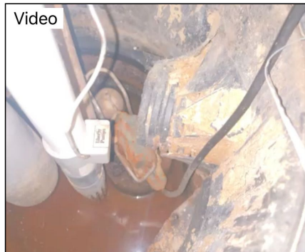
Sump pump tested ok by (lifting float)
